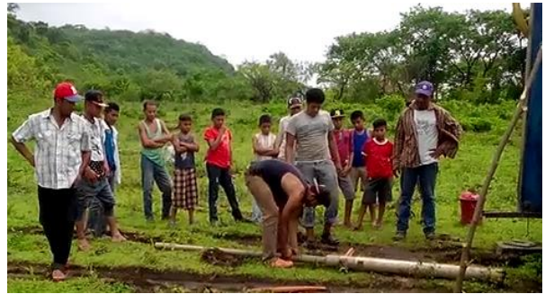
Installing the water system.
