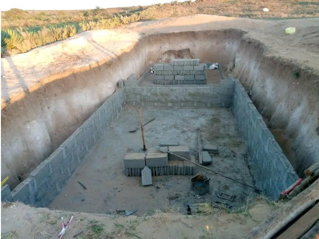
Water catchment reservoir under construction at Esanta in southern Madagascar.
