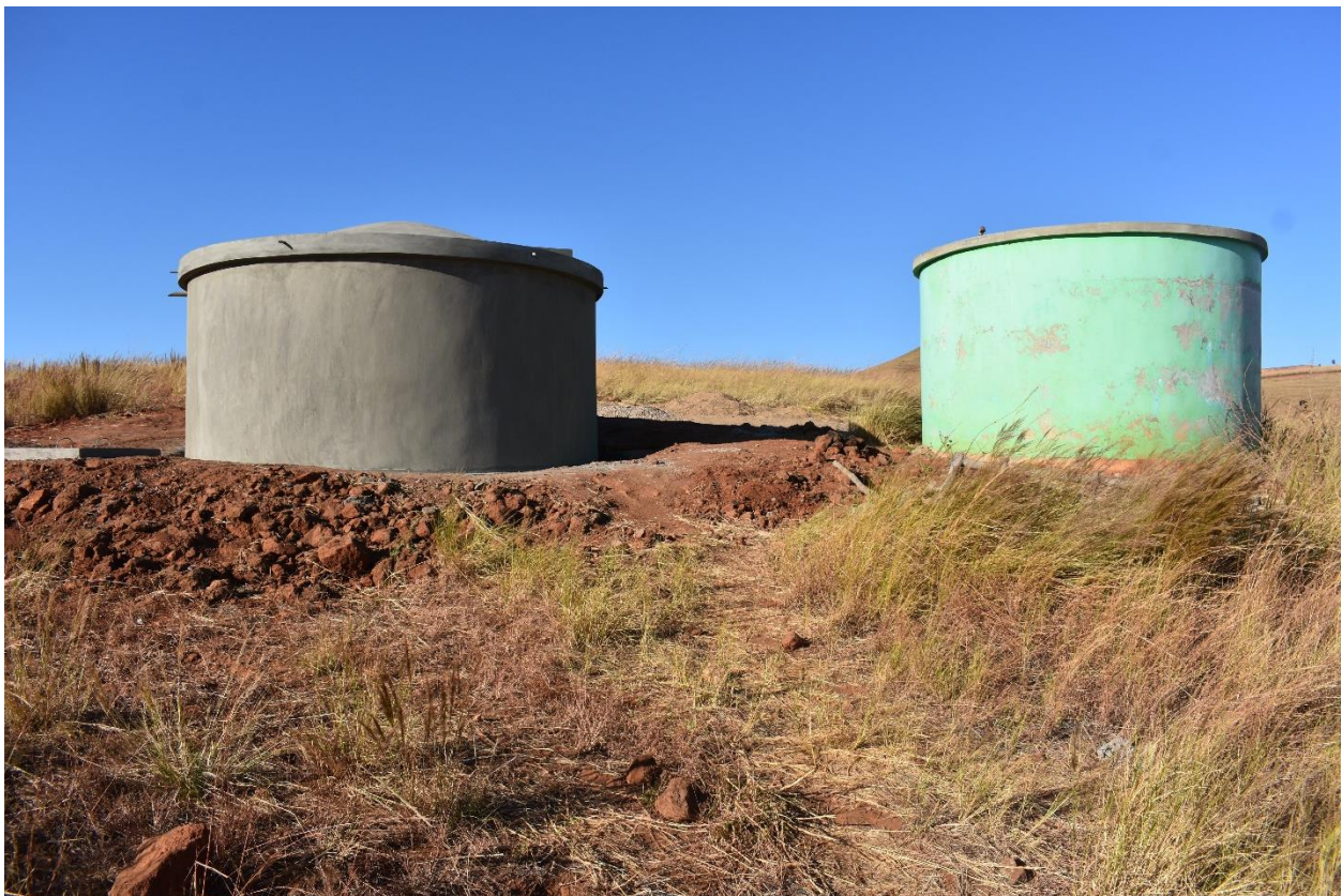
New water reservoir (on left) at the Mango Palace
