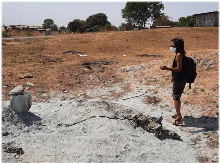
The start of a borehole that will give water to a PCOSS School
